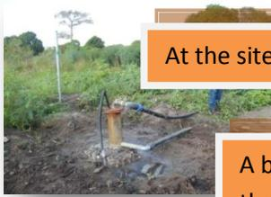
At the site an artesian well taps into an aquifer. The site has a capacity of 30,000litres/hour.
