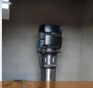
A booster pump transports water from the base station to the nearby storage tanks, which are connected to overhead tanks on a hill 7km away. The four on-site storage tanks have a capacity of 7,500litres each.
